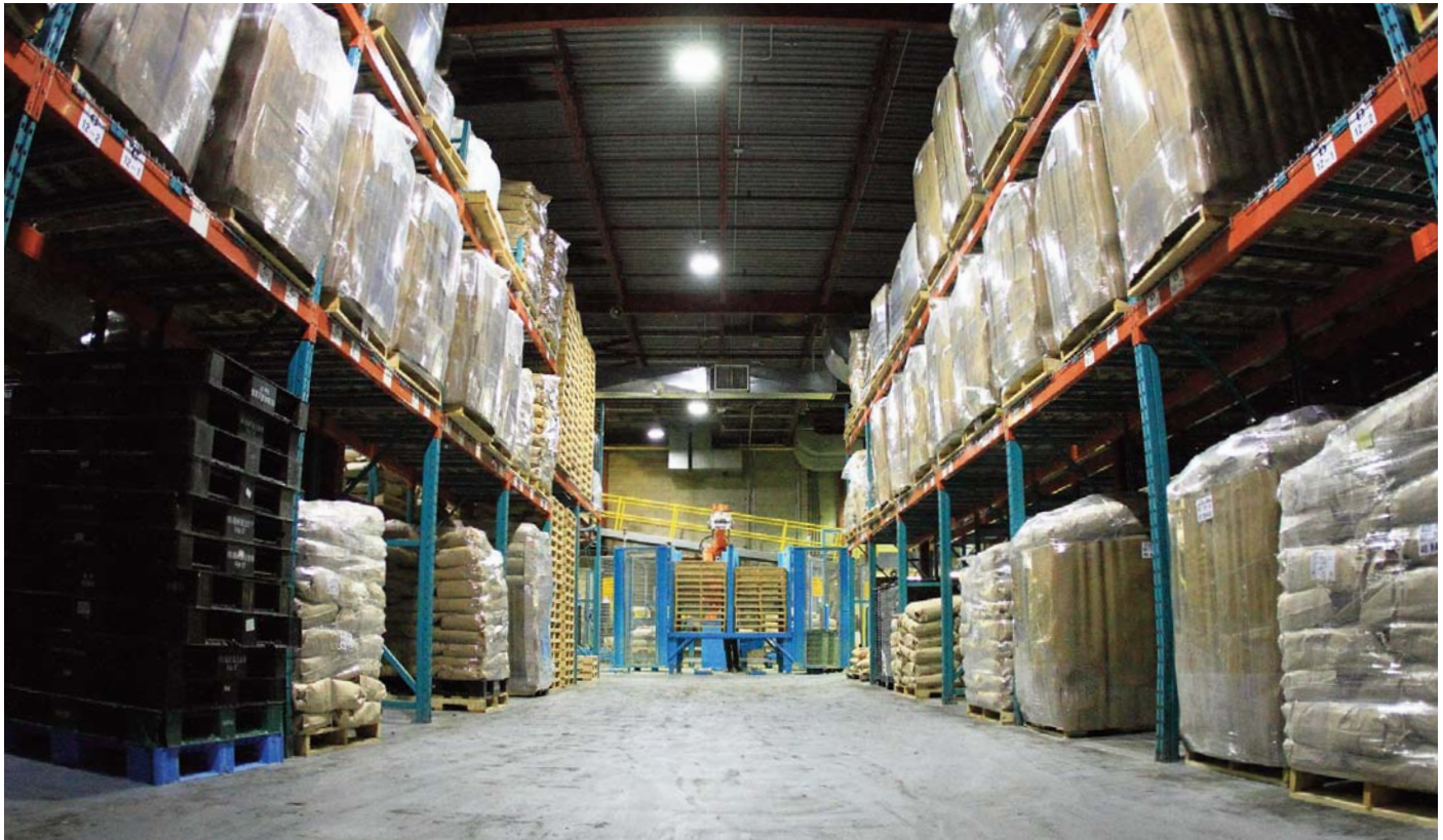
Dialight's Dialight LED High Bay Fixtures at G.S. Dunn quality control and inspection facility in Hamilton, Ontario
